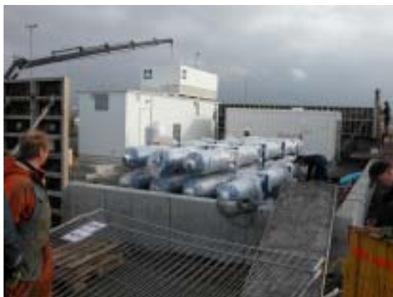
Pictures from the construction site, Skeljungur's Hydrogen production, compression and filling station, 1 st – 23 rd of March 2003.
